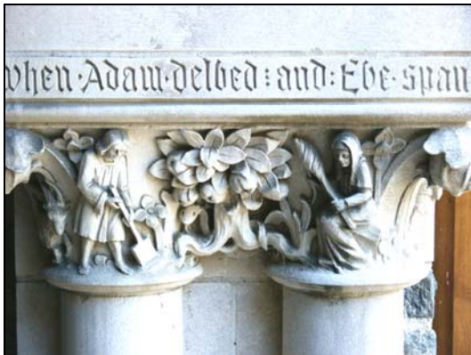
Column Detail from the Parish Hall
